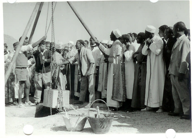
Corner stone laying by Abune Abraha
