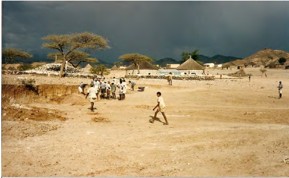
Ground preparation for new Church (1985)
