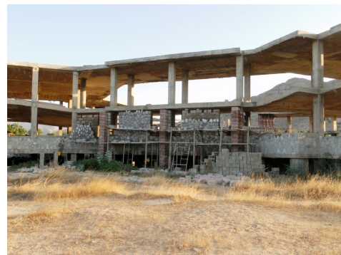
Beginning of work of the outside
