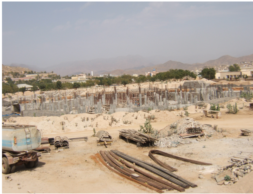
Underground being built
