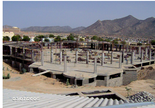
Underground covered with concrete slab
