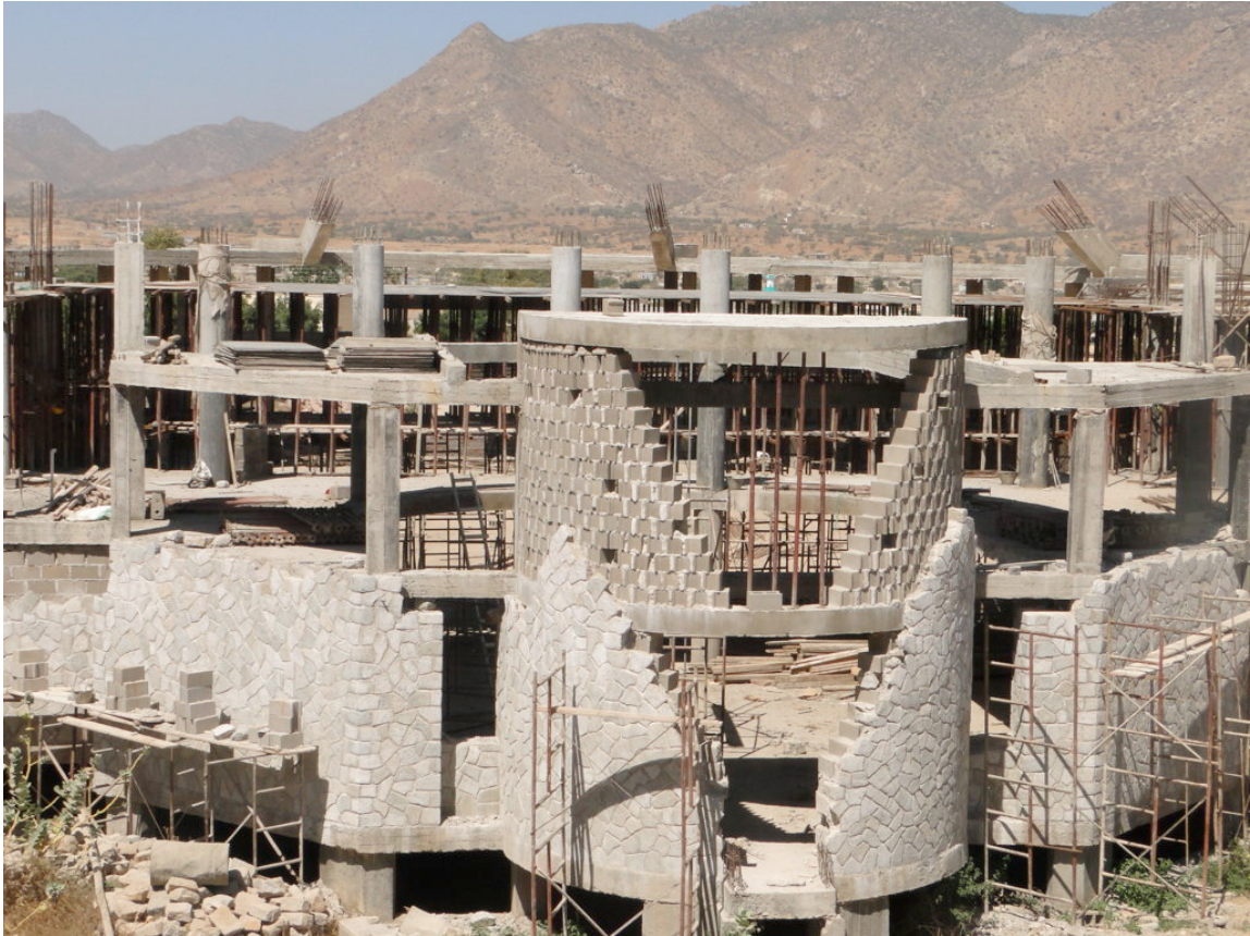
Exterior wall building process in progress
