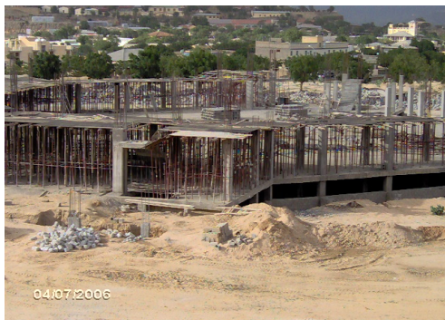
Mezzanine being covered
